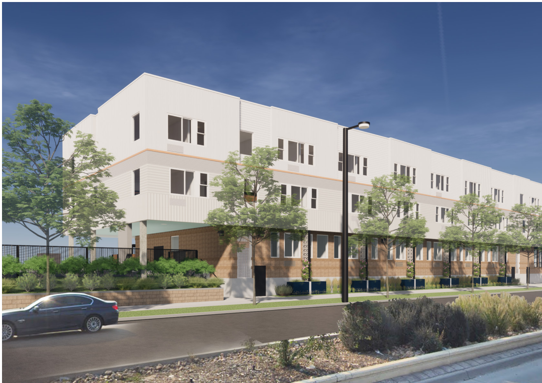
Rendering: Rhonda's Place in Denver, where permanent supportive housing units and functional layouts led to central gas DHW systems.
