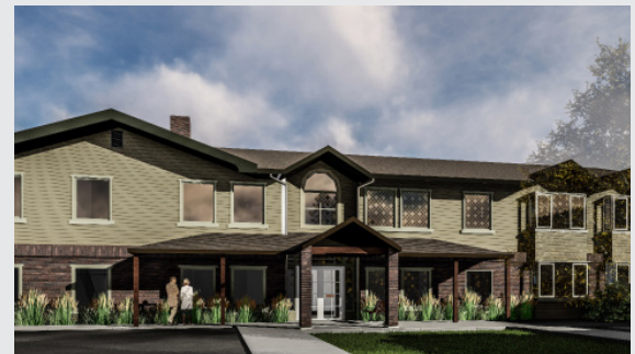
Platte River Power Authority is the utility provider for Cinnamon Park in Longmont, CO.
