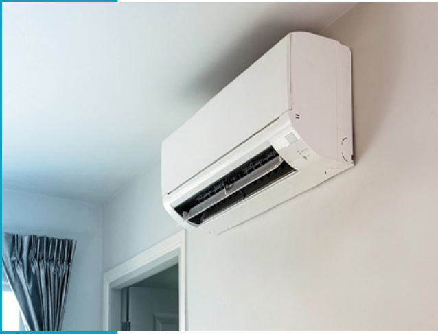
Above: Ductless Mini-Split Heat Pump
