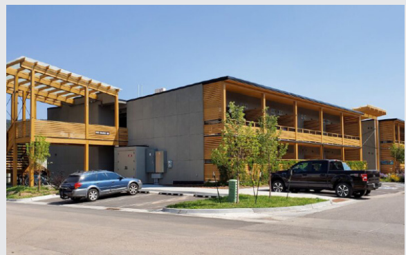
Holy Cross Electric is the utility provider for Red Hill Lofts, built in 2021, and located in Carbondale, Colorado.
