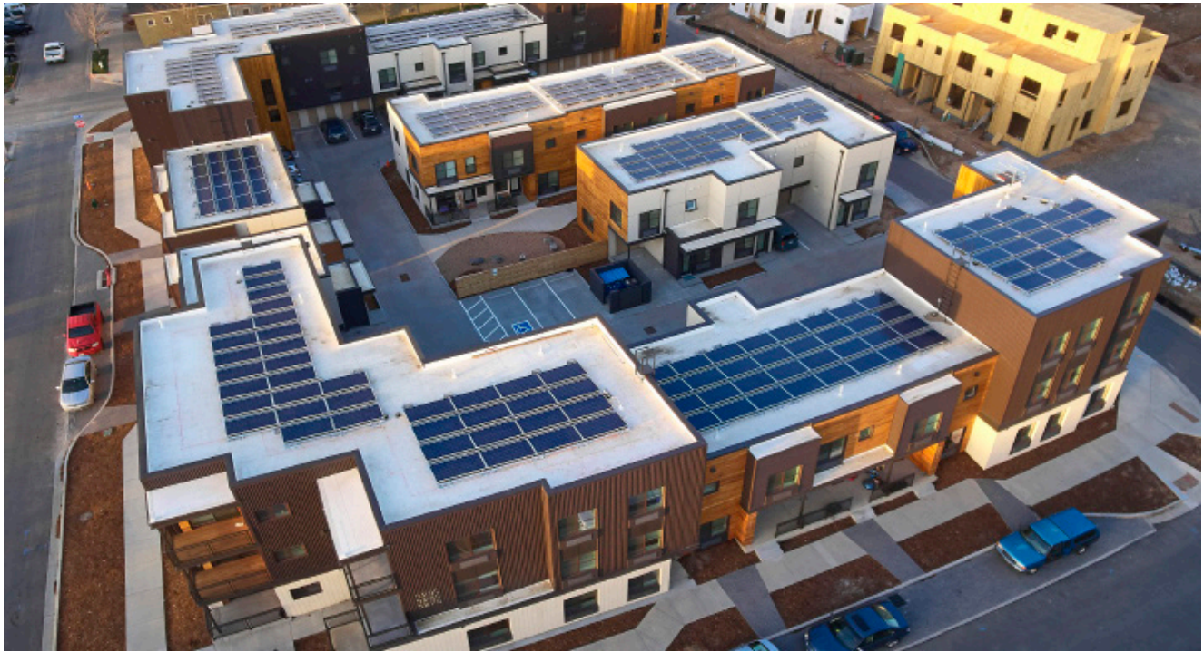
Above: Rooftop solar panels at Spark West in Boulder, CO.
