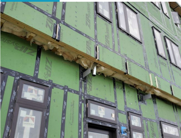
Above: Continuous Air Barrier Building Envelope
