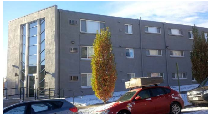
Housing & Work Connections (HAWC) Apartments
